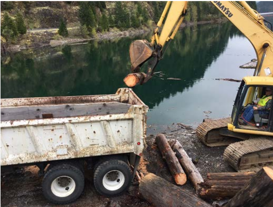
Figure 9-2. Loading Woody Debris into Dump Truck on Cougar Dam Access Road
