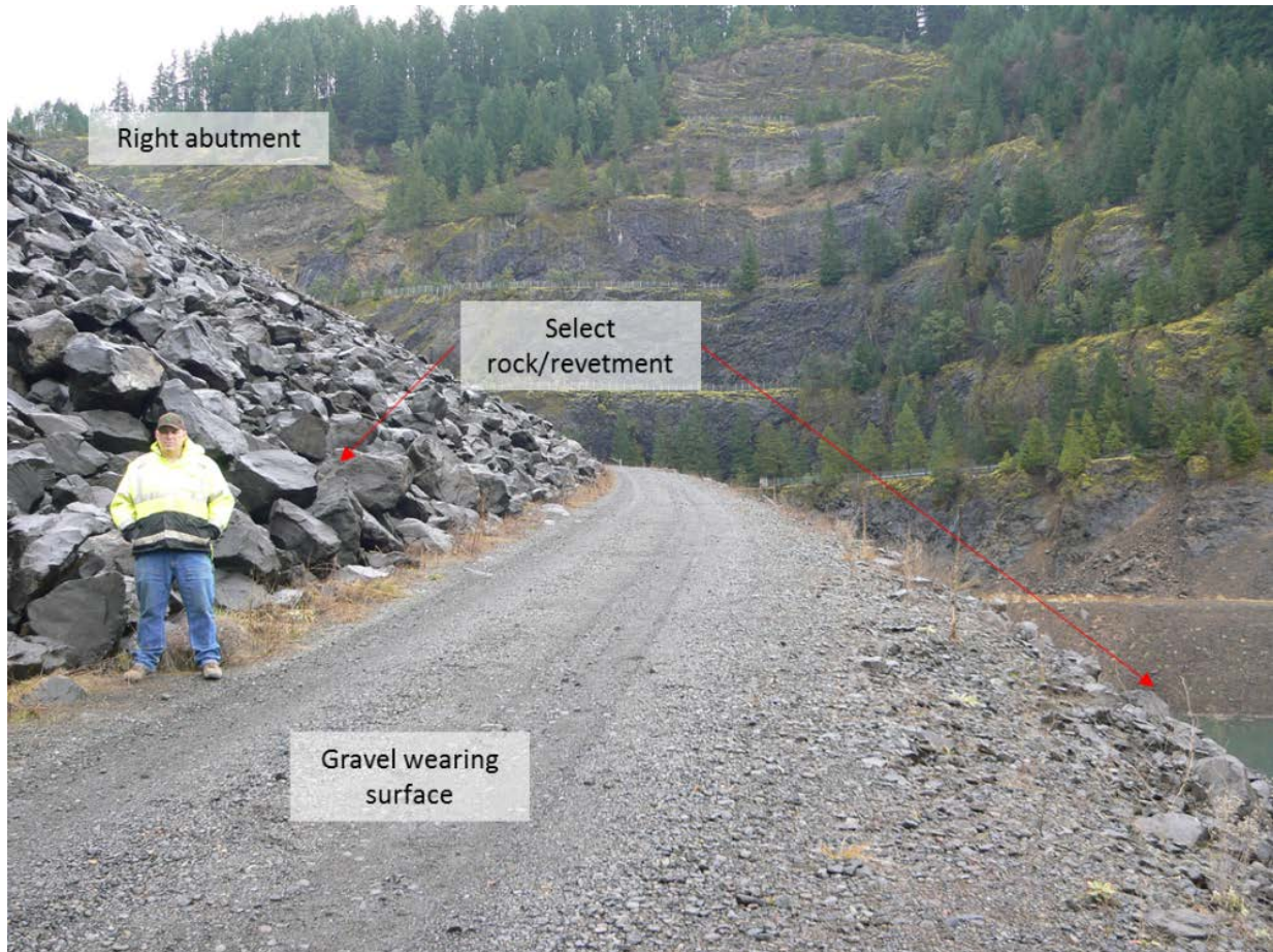
Figure 10-18. Existing Conditions Along Upstream Access Road - View to the East
