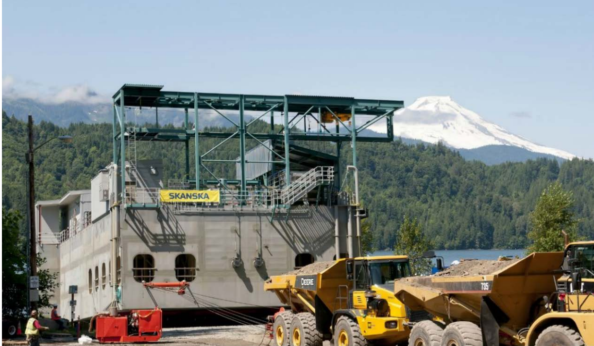
Figure 14-1. Skanska Launching the Lower Baker Floating Surface Collector with Hydraulic Dollies and Dump Trucks
